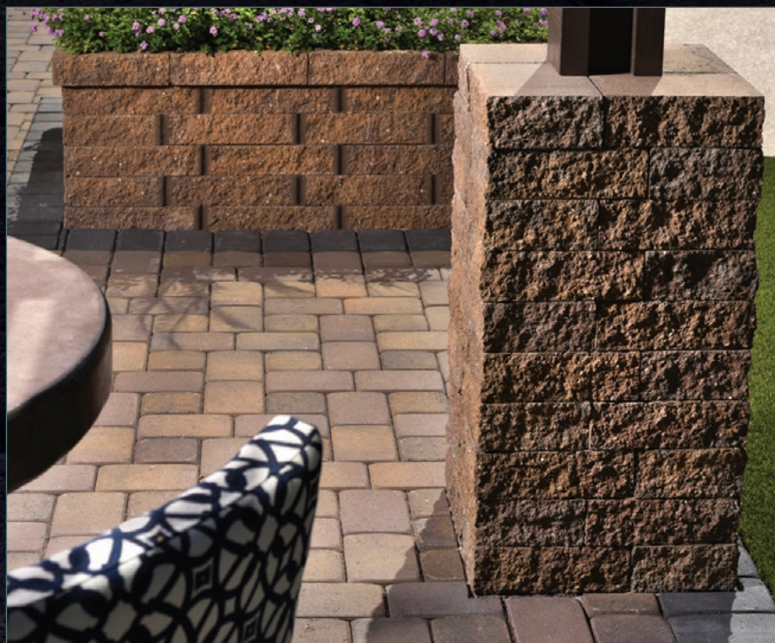
Planter – Mesa Wall with Caps Column – Mesa Wall Caps cut on location. All in : Territorial
